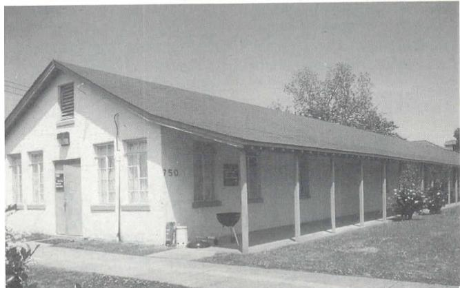
Maxwell's WWII barracks were extremely well built and adapted to the hot, humid southern climate. Like Maxwell's prewar construction, the buildings' walls were hollow-core tile covered with stucco. This material was not only fireproof and low maintenance but also provided excellent insulation. Barracks had a full-length screened porch, a feature that made humid hot summers more bearable. Most of Maxwell's WWII barracks have been substantially remodeled or demolished.
